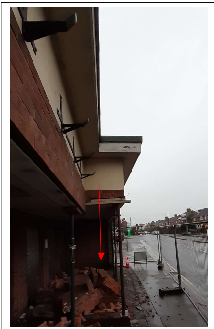
Photo No.2 – View of Demolished Pier
