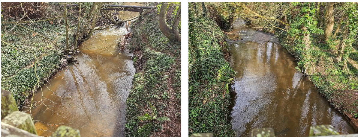
Figure 17: Back Stream crossed (left image is looking upstream (south) and right image is looking downstream (north)).
