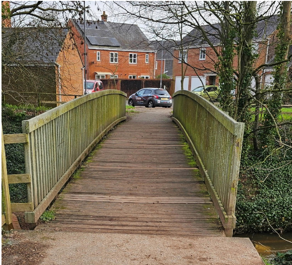
Figure 6: West looking east along bridge.
