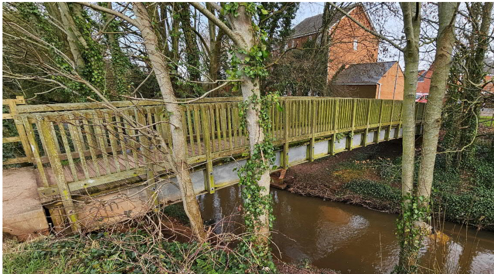
Figure 2: Bridge southern elevation.
