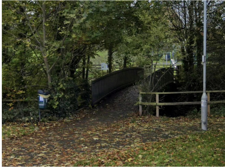
Figure 16: Western approach (google image).
