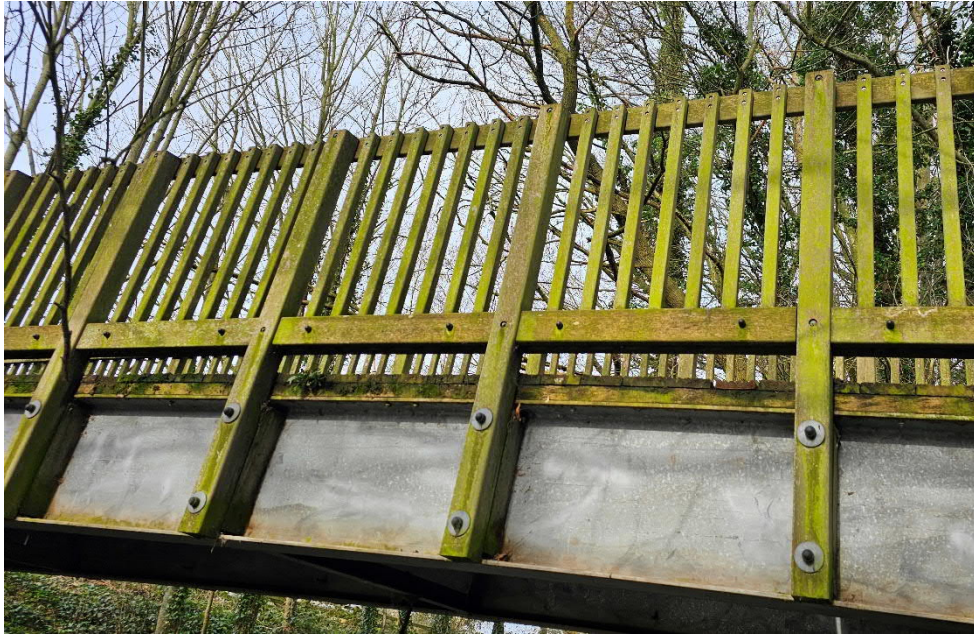
Figure 10: Parapet arrangement.
